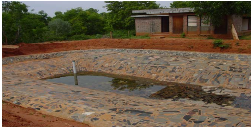
RAINWATER HARVESTING POND
