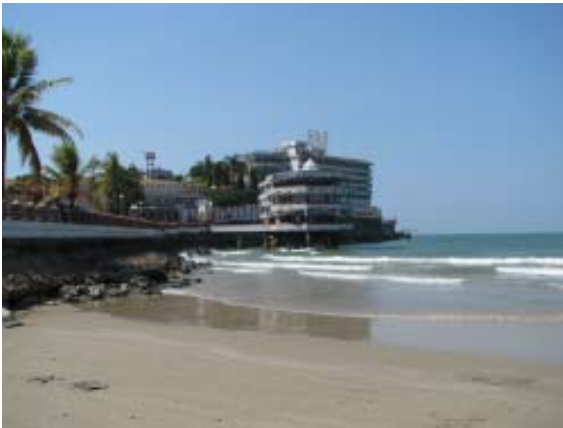
CRZ violation, Murdeshwar, Uttara Kannada, Karnataka Photo: Sudarshan Rodriguez
