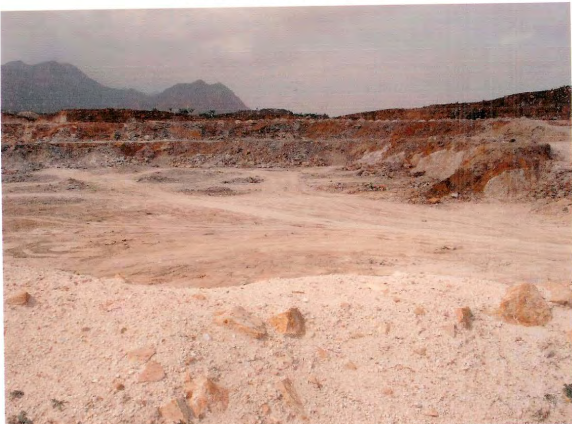
Photo plate No.6: Large Mine pit serving as a recharge reservoir in Thandiberi mines
