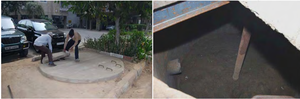
Figure.21. AR structure constructed at Som Vihar Apartment, RK Puram, New Delhi
