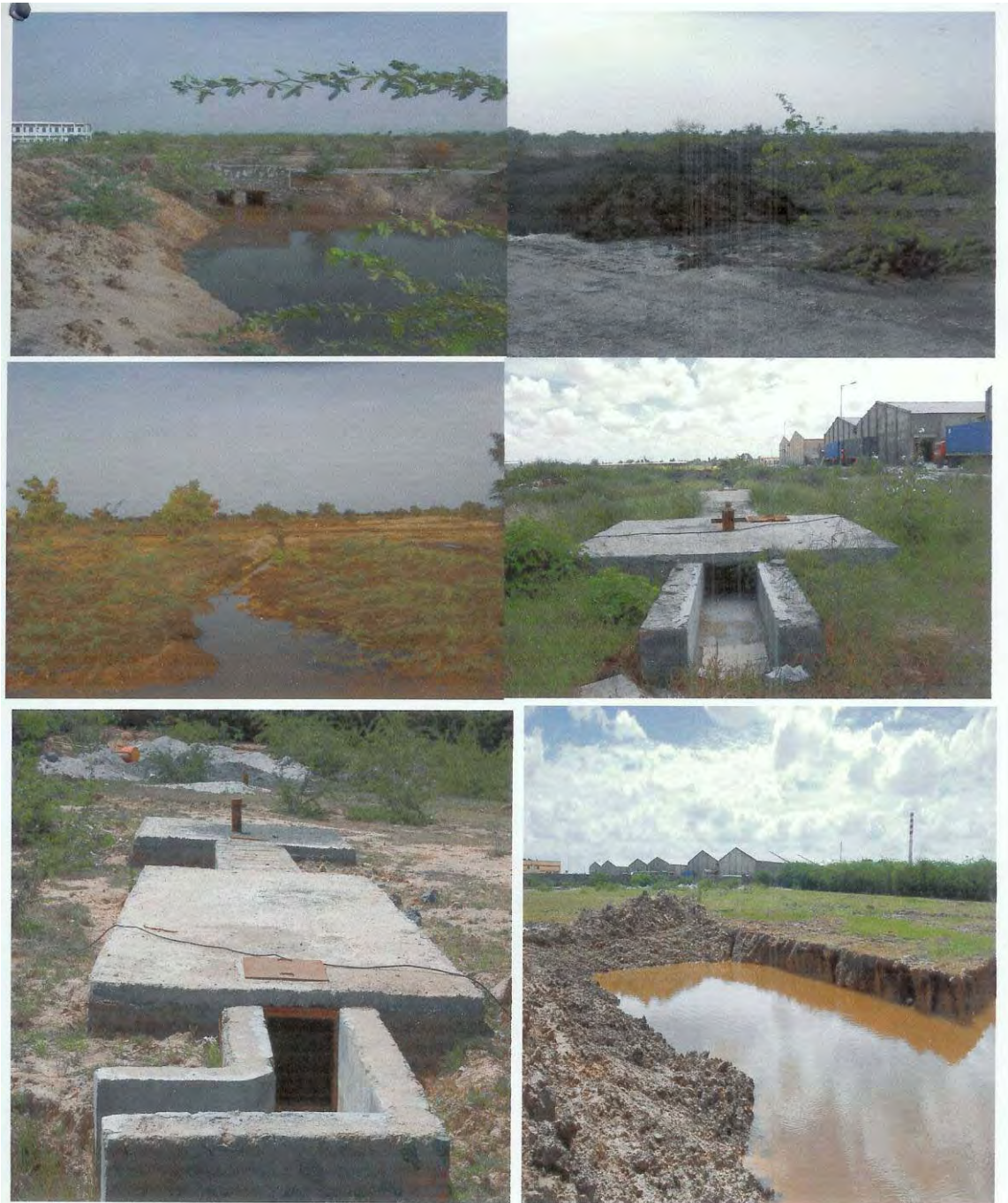
LOCATION/ CATCHMENT AREA OF RAIN WATER HARVESTING STRUCTURES
