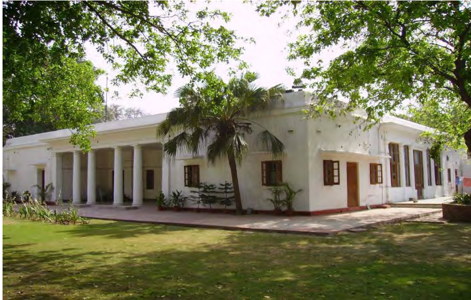
Figure. 16 Rain Water Harvesting and Artificial Recharge to Ground Water at Gandhi Smriti Bhawan, Tees January Marg, New Delhi
