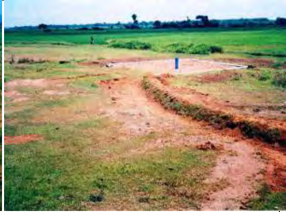
B. Barkatia Watershed – Recharge Pit with Bore Well
