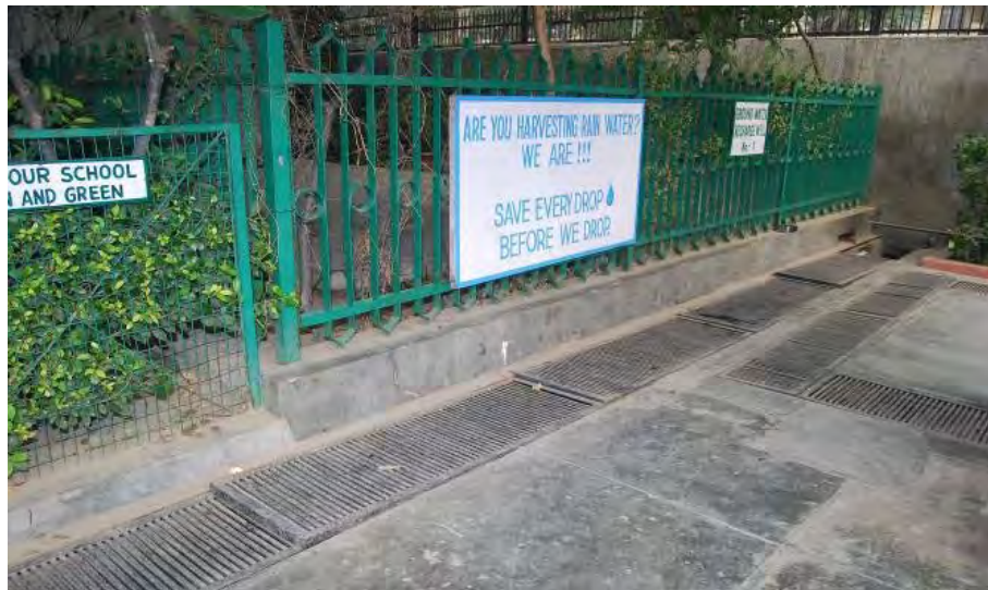
Figure.20. AR structure constructed at Mira model school, Janakpuri
