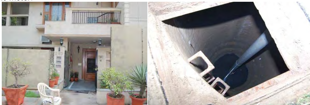
Figure.23. RTRWH & AR structure constructed at Defence colony, New Delhi
