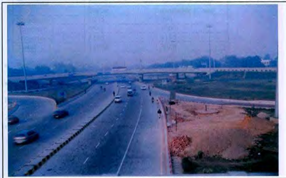
Figure.15 Artificial Recharge Structure at AIIMS Fly-over
