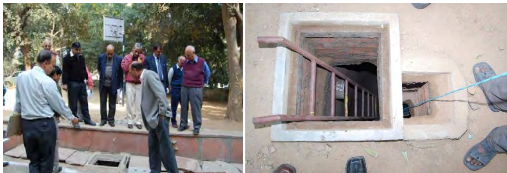
Figure.22. AR structure constructed at Resident Welfare society, Alaknanda New Delhi
