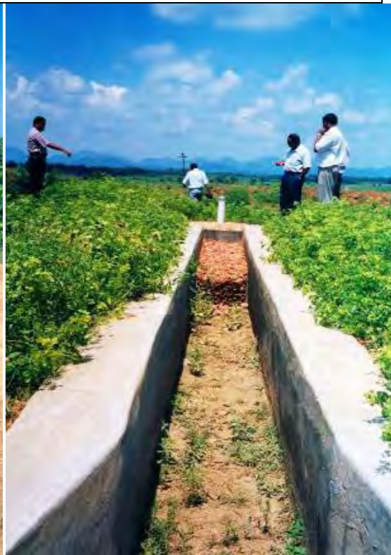
D. Barkatia Watershed - Trench with recharge Bore
