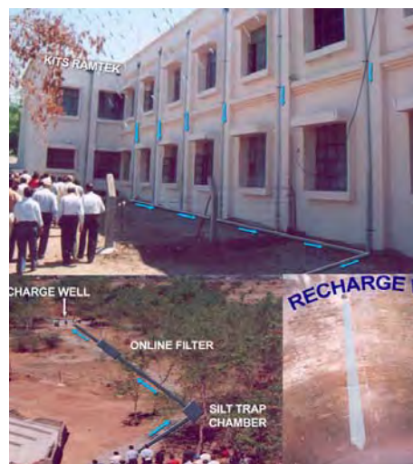
Figure.36. AR structures shaft with recharge well.
