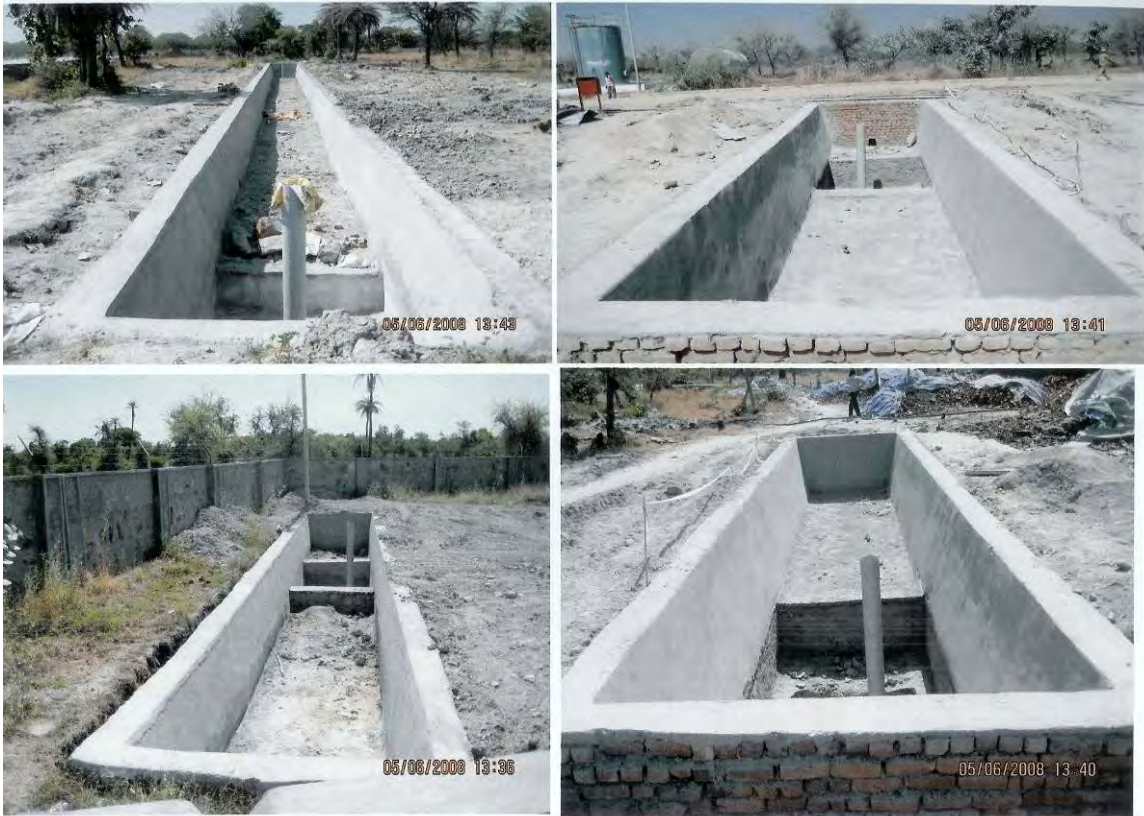
RAINWATER HARVESING STRUCTURES
