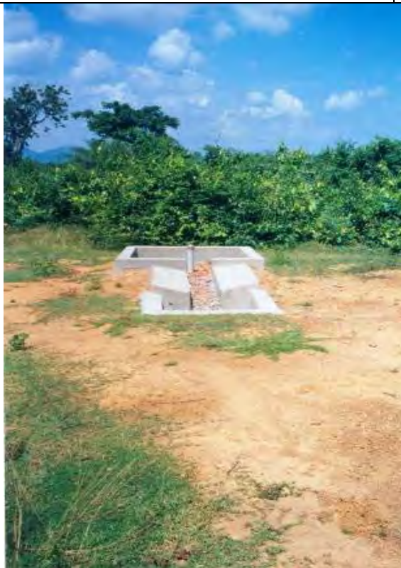
C. Barkatia Watershed – Recharge Bore
