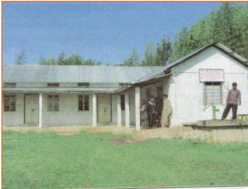
Laitkseh Govt. L.P. School, Mawryngkneng Block, East Khasi Hills School Building has been extended over the tank
