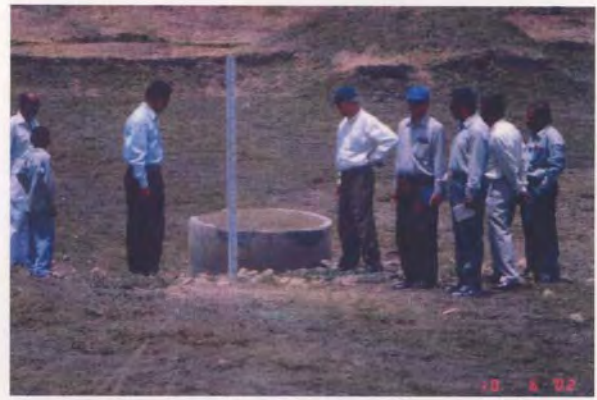
Figure.30 Recharge Shaft at Mendkichak District Dewas
