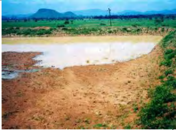
A. Barkatia Water Shed – Percolation Tank
