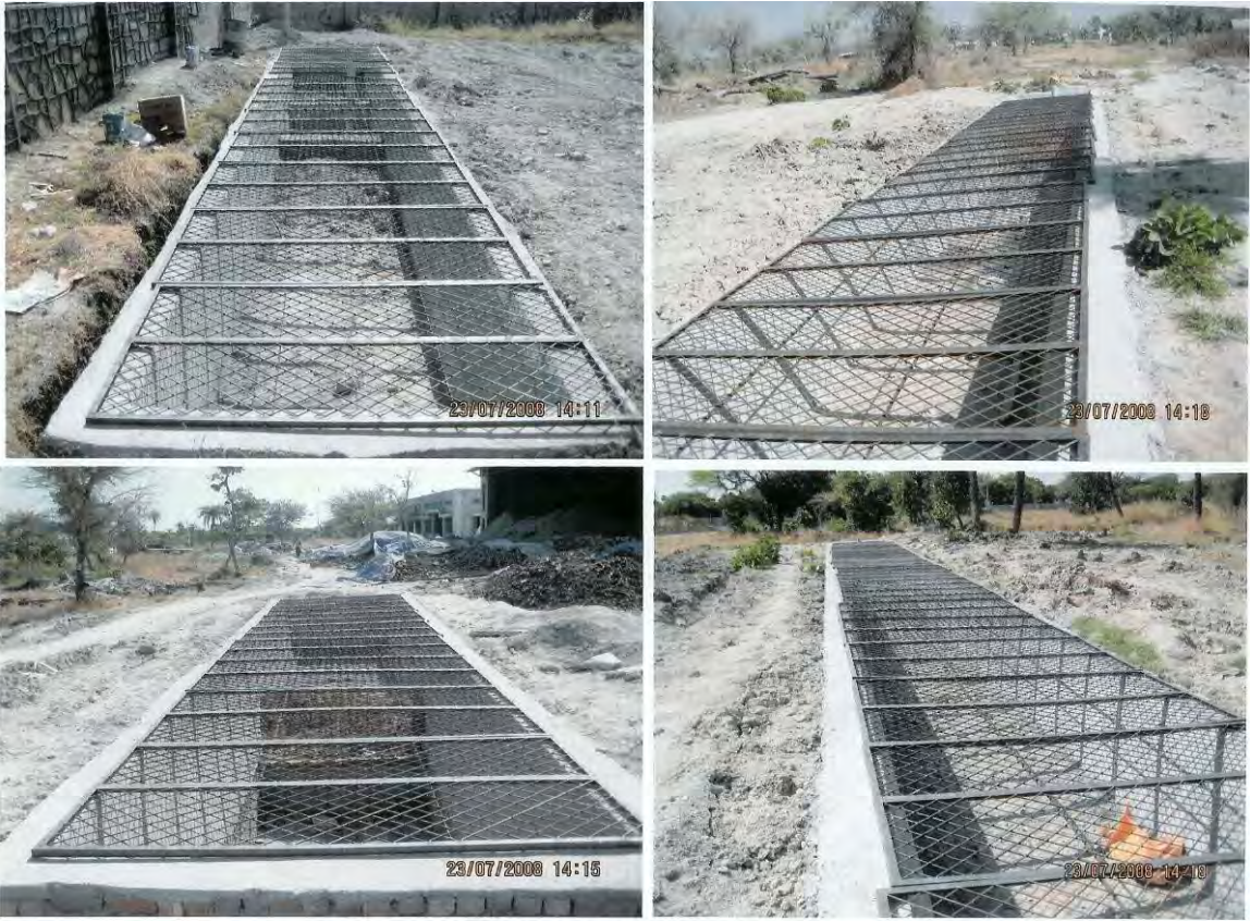
RECHARGE TRENCHES WITH INJECTION WELLS
