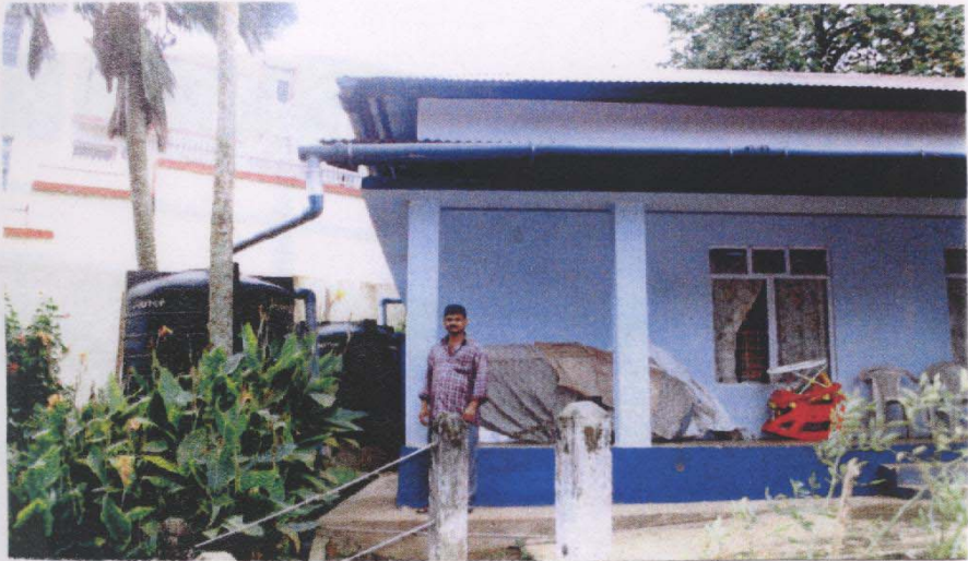
CIRCUIT HOUSE, LABAN, SHILLONG
