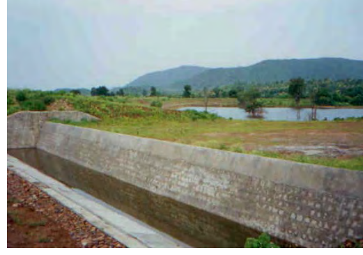
Fig.34b.Percolation Tank at Benoda
