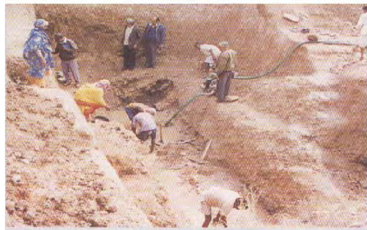
Figure.26. AR structure- Subsurface dyke under construction at Burhanpur District, M.P.
