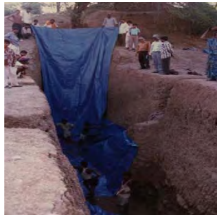
Figure.28. Subsurface Dykes at Londri Nala, District Dewas
