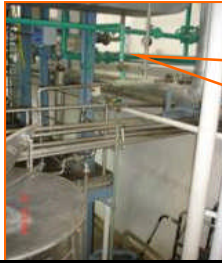
Fresh water line disconnected and connected with Cooling water
