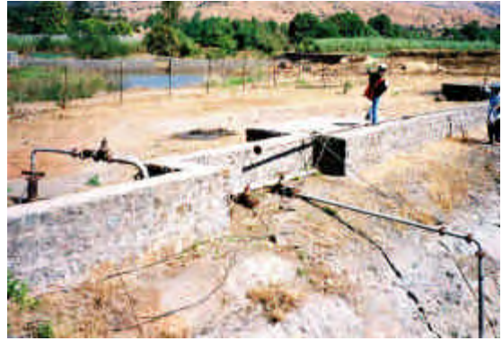
Water being pumped from bore well (above) and is stored in the dug well (below) during the summer period
