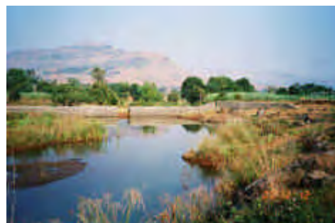
Check dam in Hadashi from which, lands along the river, are irrigated using diesel engines
