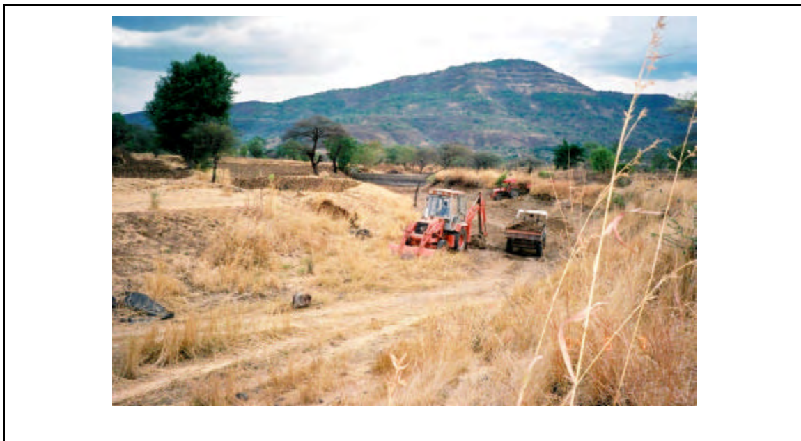
Check dam CD3 was desilted in May 2004. Some 7 mm of silt accumulates in the structure every year.
