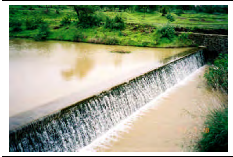
Check dam CD2 in Chikhalgaon, overflowing during the monsoon.
