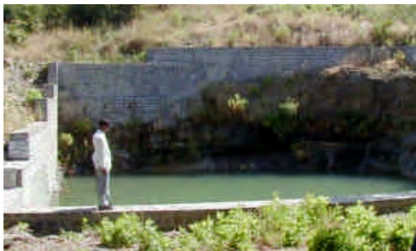
Spring tank in Bhalgudi...
