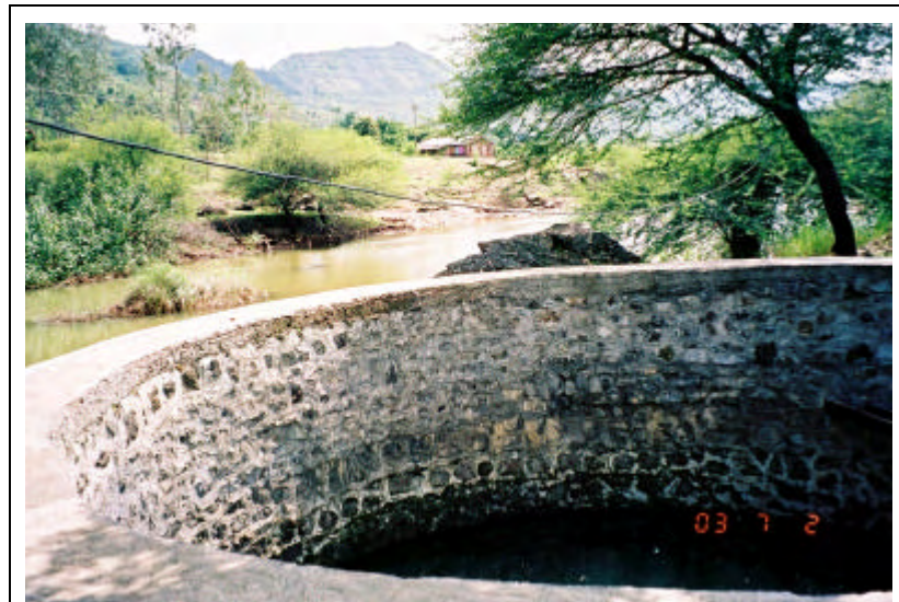
Dug well CH1, with river in the background; the well supplies water to Chikhalgaon village.
