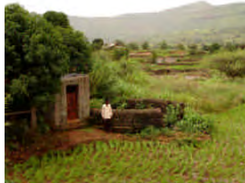
Pumping well for the scheme
