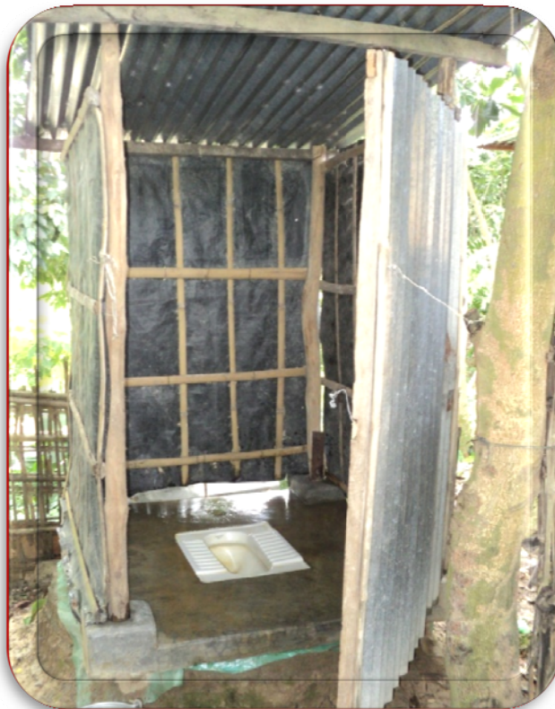
LOW COST TOILET, SOUTH TRIPURA
