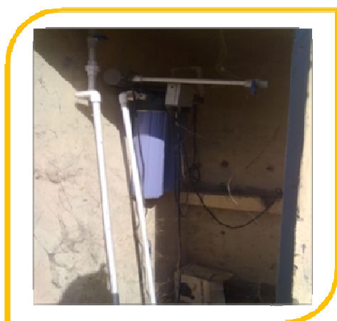
Water connection not given to the over head tank
