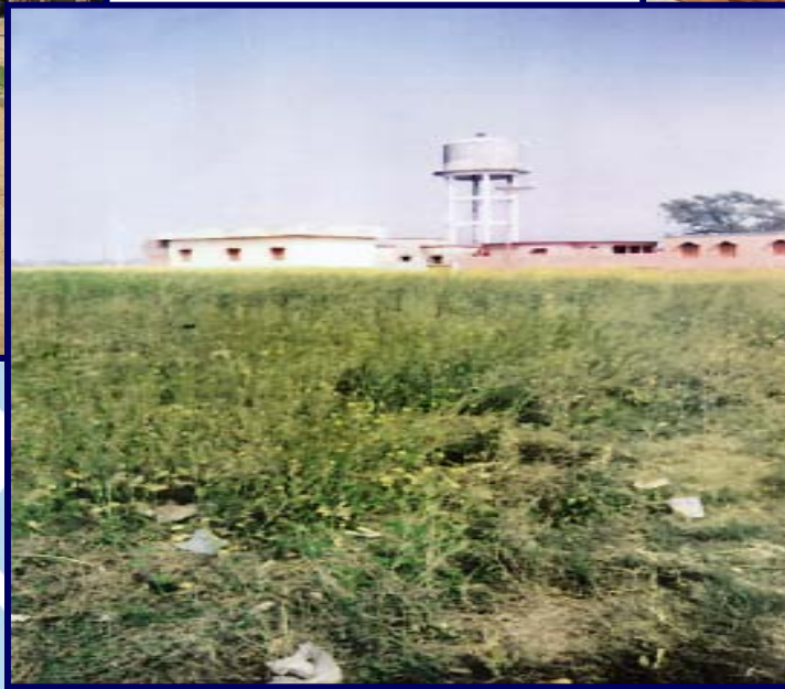
DEFUNCT OVERHEAD TANK TO TAP SAFE AQUIFER
