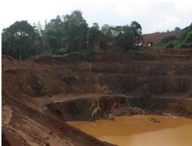
Pumping of water from Cavrem Sheikh Salim mine, severely lowering groundwater table in the village. Photo with thanks from: Sebastian Rodriguez, Mand Goa
