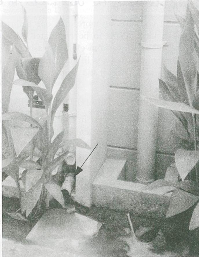
**Picture 12.5** Here a separate gully connected to the treatment bed has been provided outside the ducting and the grey water directed into it using two PVC elbows and an extension pipe. These extensions were fixed without using any jointing fluid, so that, if required, they can be removed and the grey water can go straight into the gully below connected to the man hole chamber in front.
