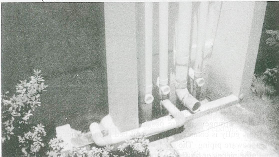
A simple inexpensive arrangement to divert the grey water to the treatment bed would be to rig up a portable piping system shown in Picture 12.8, made from a plastic mug and a PVC or polythene garden hose.
