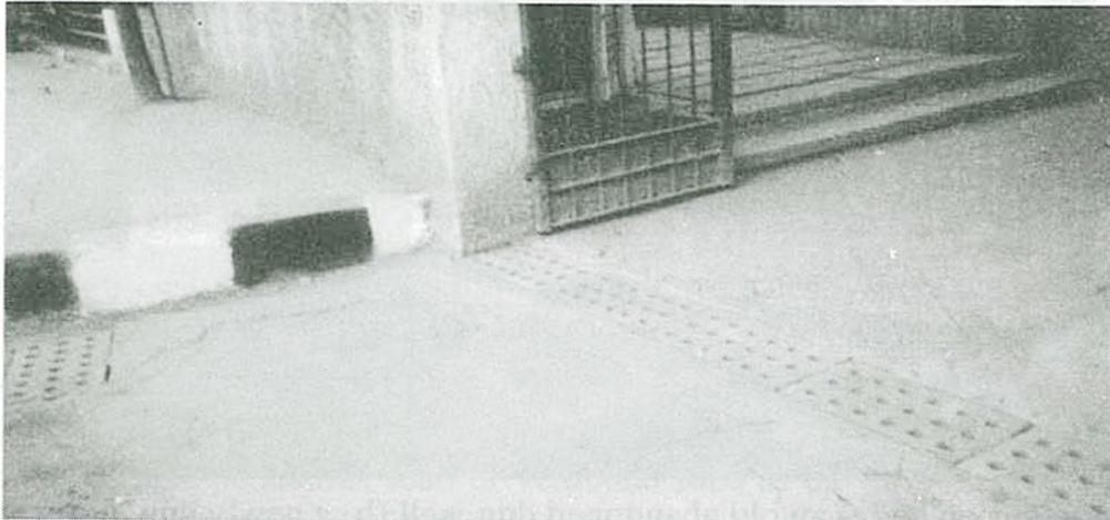
**Picture 7.13** This is a complex of 48 flats in two blocks opposite each other. The trench has been located inside the premises, away from the gate and can be seen just behind the car. It spans the stretch between the two blocks. This has been done because the road level is slightly higher and road rainwater mixed with sewage tended to enter the premises during monsoon. Additionally speed breakers were also put near the gate to prevent the ingress of road water into the premises.
