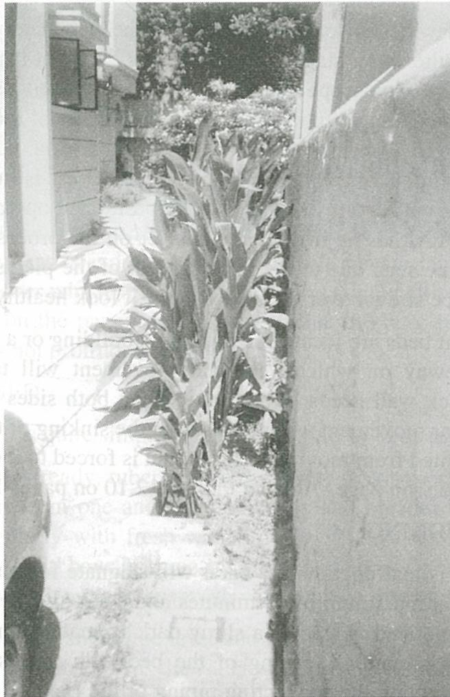
**Picture 12.10** The 1ft bed was close to a compound wall on one side and at the edge of a paved driveway on the other. Therefore walls were put on both sides. You can see the dried parts of the plants fallen on the ground. If these are not removed, free flow of grey water over the bed is hindered. Note that the level of the treatment bed is lower than the level of the driveway..
