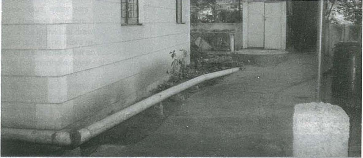
**Picture 7.5** The rainwater pipe is given a bend inside the dug well (as seen ) so that the rainwater flowing in with some force hits the side of the well, loses its momentum and flows down the wall, without disturbing the water column in the well. This acquires value in the dry season when the water column is less and turbulence may result in muddy water being pumped up. All these pictures are from the author's own colony.
