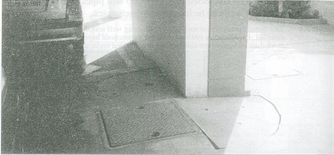
**Picture 7.7** Another view of the dug well inside the building. The solid line demarcates the well and the dotted line the manhole cover.
