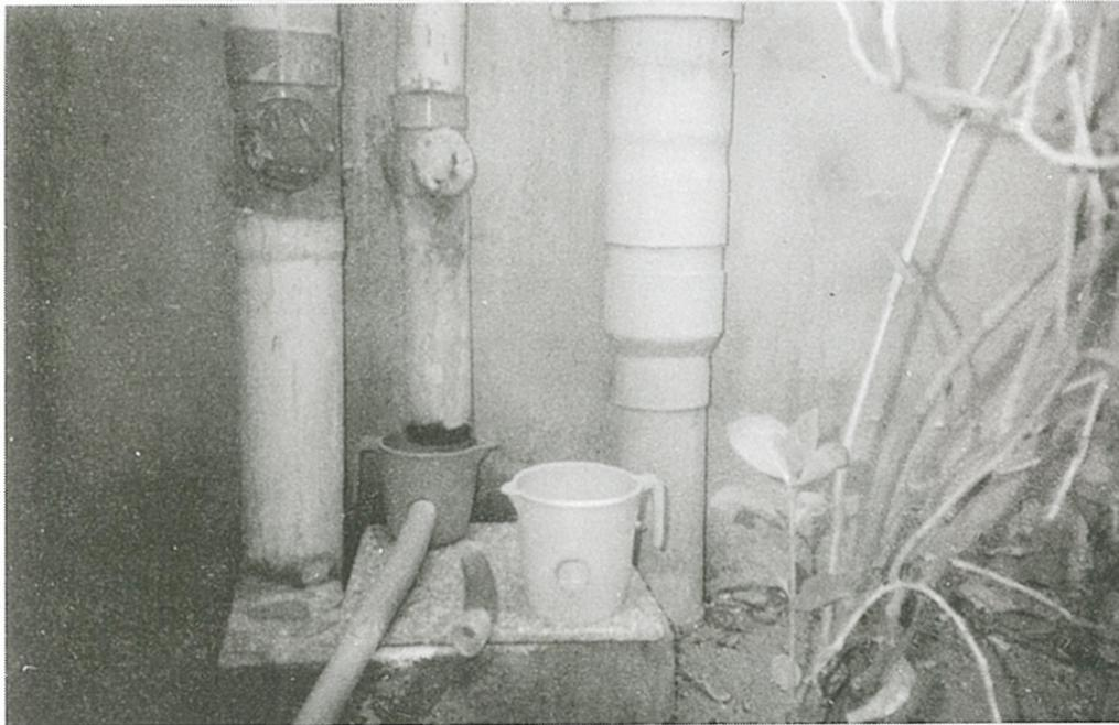
Such an arrangement is indeed inexpensive and can be laid even across a paved driveway over which vehicles may pass by simply chipping off a semi-circular channel on the paved driveway such that the hose just fits in to the channel and does not protrude above ground.
