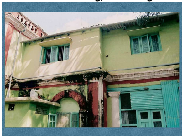
Rainwater Harvesting at City Municipal Council Building, Chitradurga
