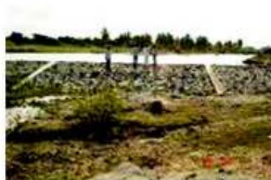
The Check Dams and Water Ponds constructed to harvest Rainwater
