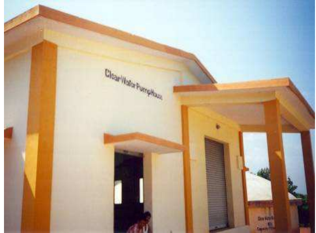
Clear water Pump house
