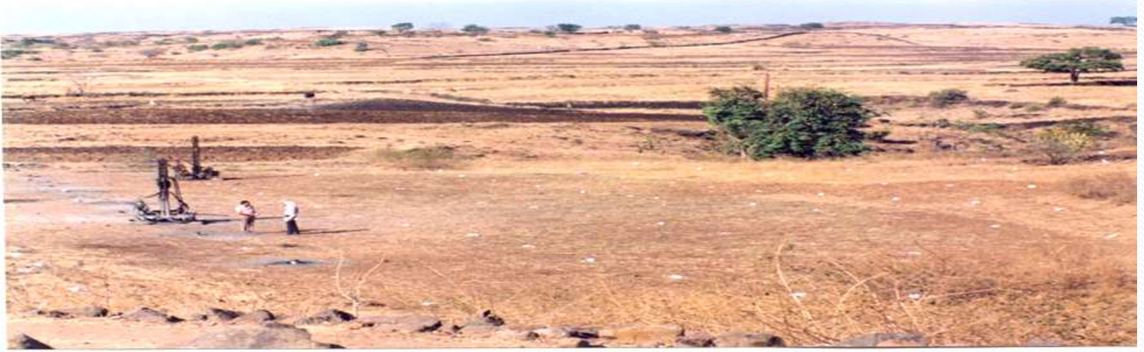
▲ DRILLING BORE HOLES FOR BBT APPLICATION
