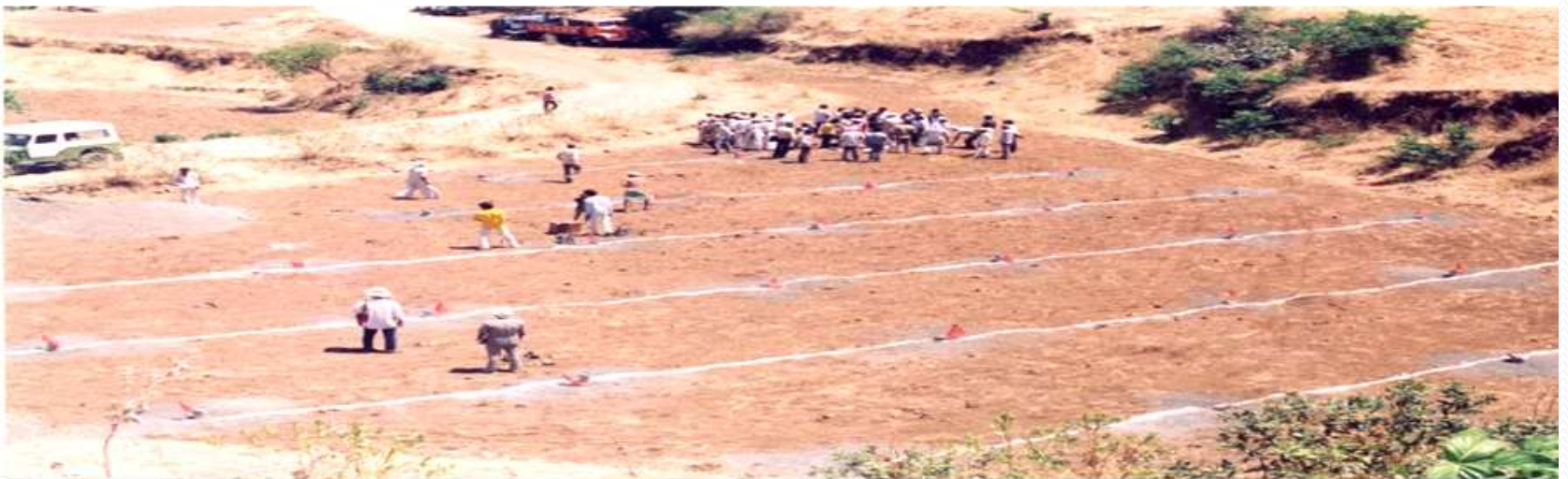
▲ SAND STEMMING & EXPLOSIVE PLACEMENT
