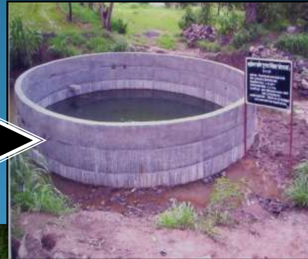
Deepening of well
