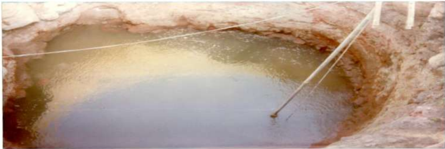
▲ AFTER JW BORE HOLE BLASTING (NOTE RISE IN WATER LEVEL)
