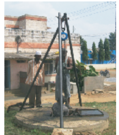
Desludging of Biogas Reactors
