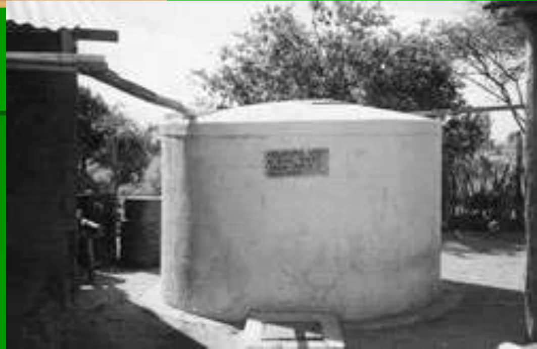
Tank in rural areas
