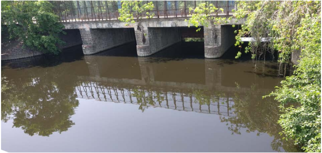
Figure 5: Hindon Cut Canal
